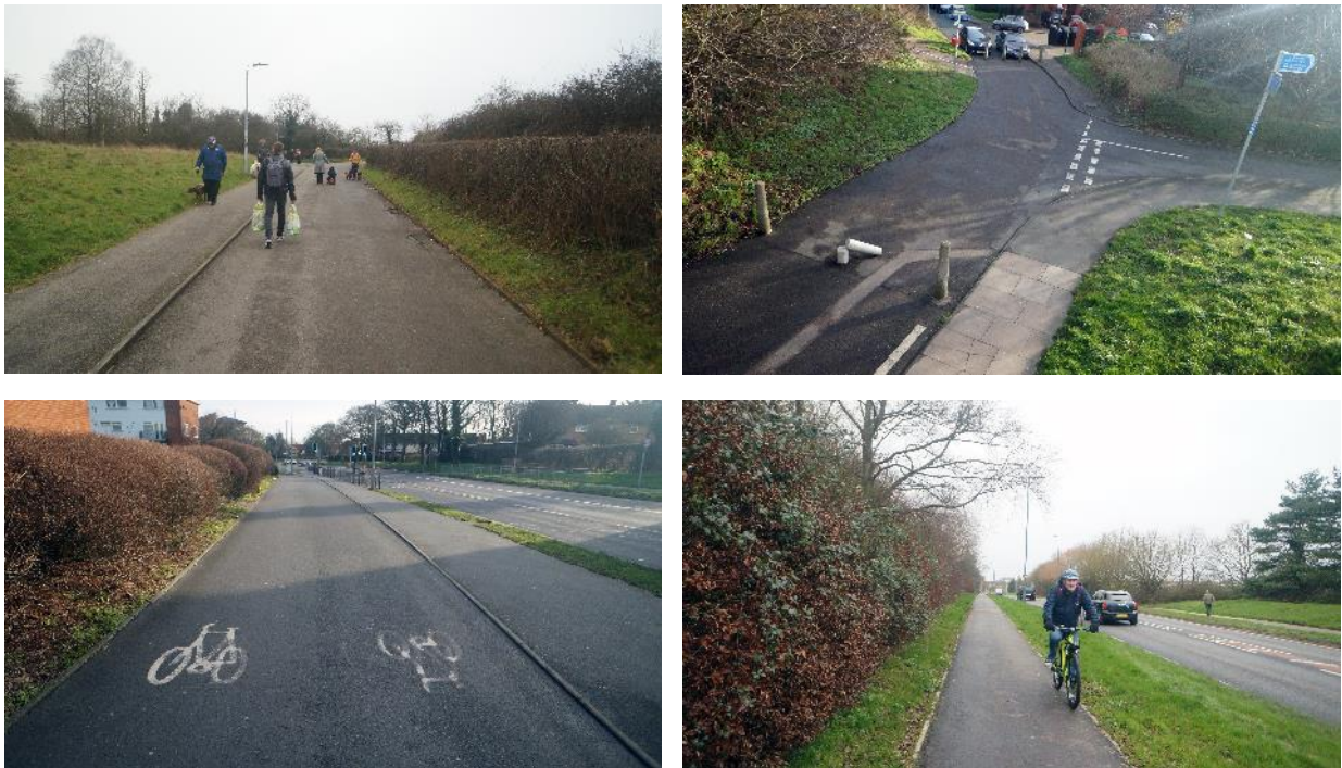
Figure 1-2: Examples of Harlow’s existing walking and cycling routes: Traffic-free route (Harlow Fields), Grade separated walking and cycling route (First/Fifth Avenue), Bi-directional cycle track (First Avenue), Shared use track (Southern Way)
