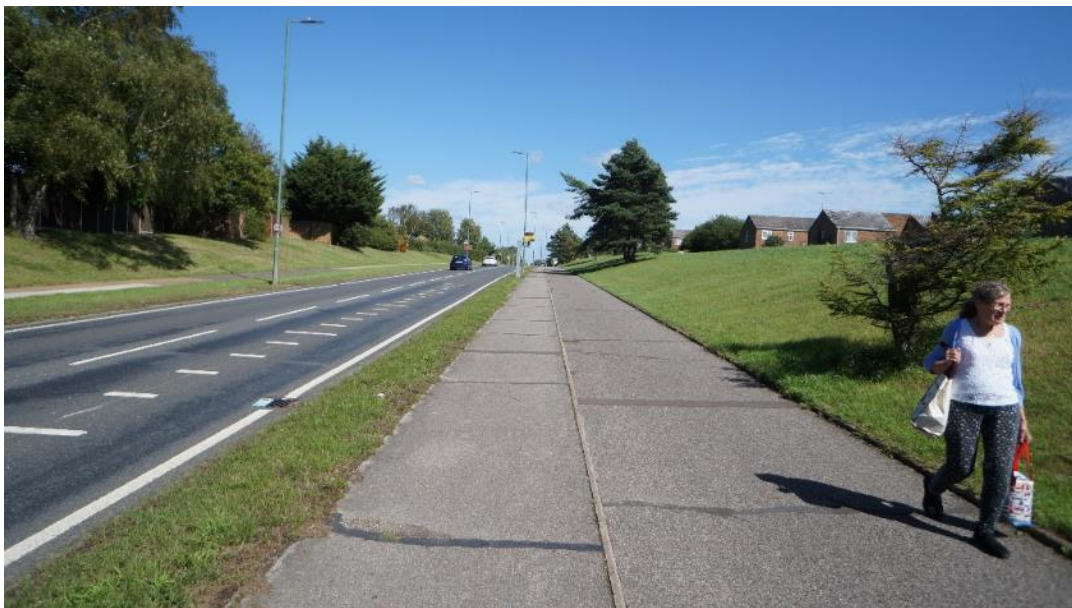
Figure 3-4: Protected cycle track and footway alongside Second Avenue
