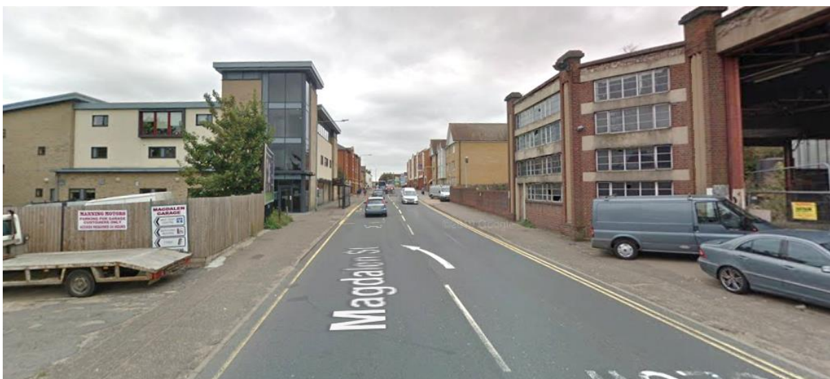
Figure 3 - A134 Magdalen Street Looking West
