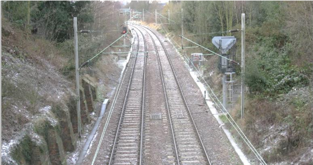
Figure 7 - View from Brook Street Bridge Looking East
