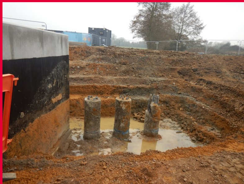
Above left: Reinforcement in the bored pile. Above right: Excavated to the formation level of the retaining wall with the top of the piles to be broken to the correct level.
