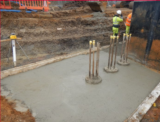
Above left: Blinding concrete completed ready for next phase. Above right: Site following recent downpour.
