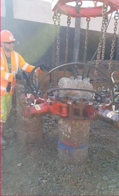
Above left: Pile cropper removing the top part of the pile. Above right: Placing of blinding concrete in progress.
