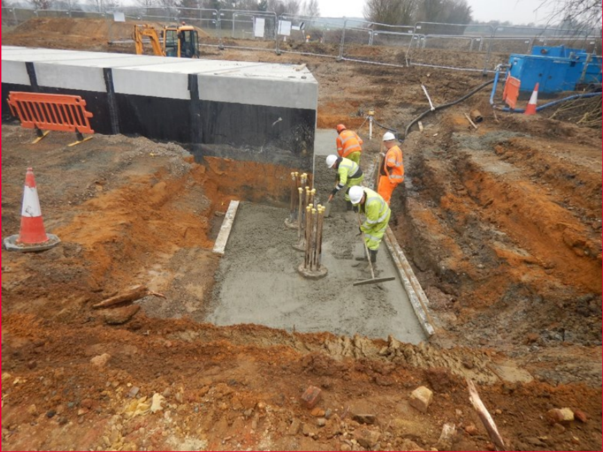
Above left: Pile cropper removing the top part of the pile. Above right: Placing of blinding concrete in progress.
