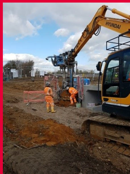
Above left: Reinforcement piles ready for installation. Above right: Piling operation temporarily stopped to allow an extension to the drilling system to be installed and the clearing of material to take place.
