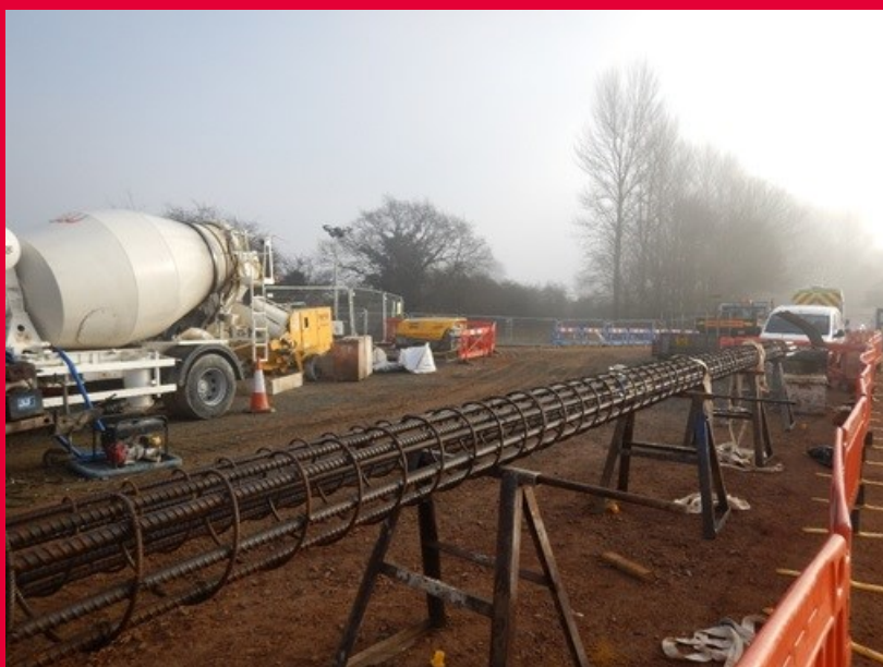
Above left: Reinforcement piles ready for installation. Above right: Piling operation temporarily stopped to allow an extension to the drilling system to be installed and the clearing of material to take place.
