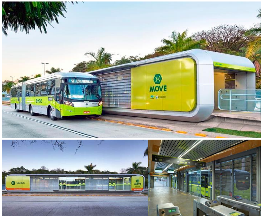
Figure 2-2: BRT stop in Brazil – the bus stop features glass and perforated plates as enclosures and uses efficient internal ventilation and lighting to create an easily maintained and pleasant space for commuters. Source: Inhabitat
