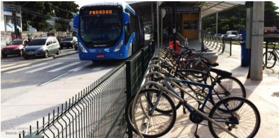
Figure 2-5: BRT station with cycling parking in Rio de Janeiro, Brazil Source: ITDP Brasil
