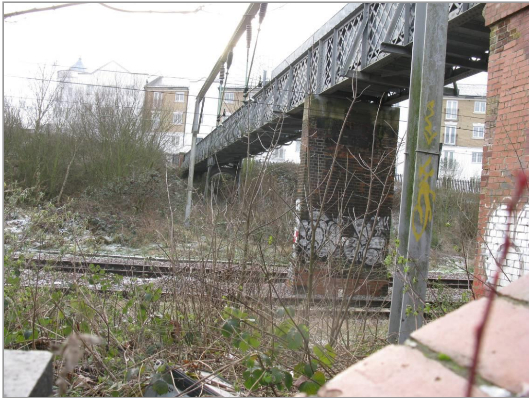
View of footbridge looking to the South
