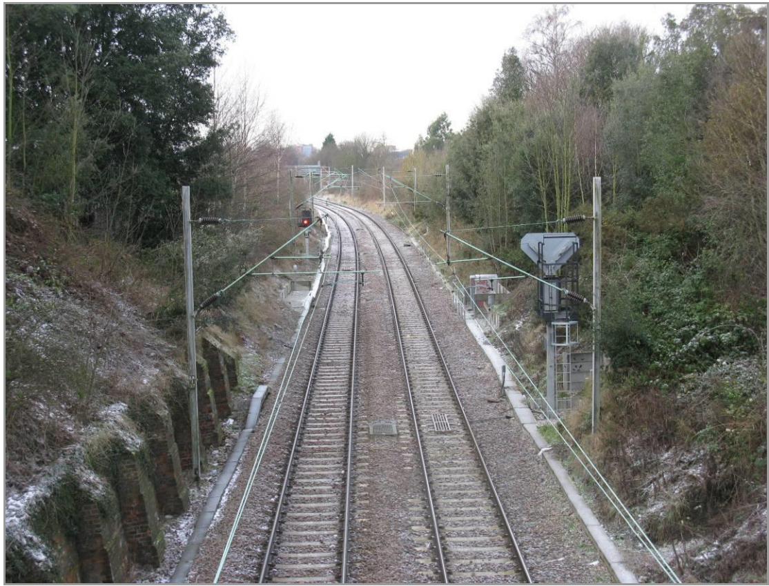
View from Brooke Street Bridge towards Hythe
