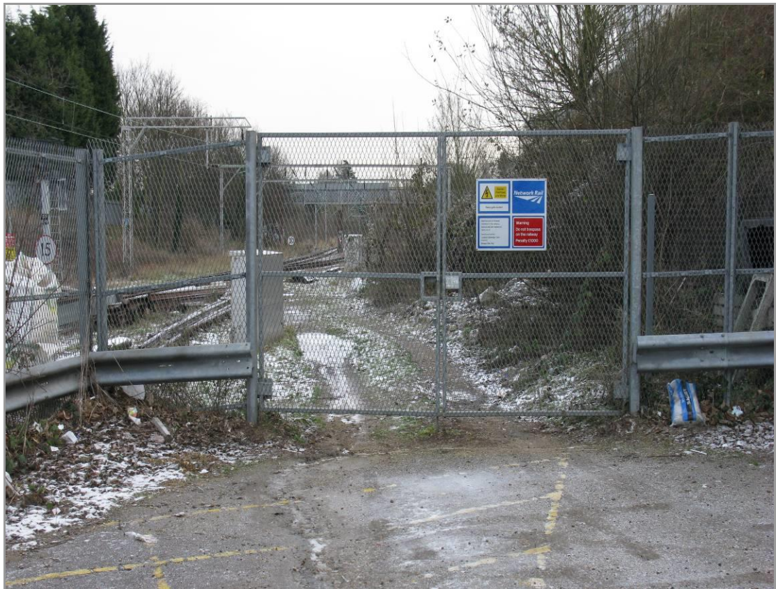
View from Station Car park towards Hythe
