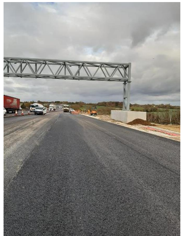
Gantry installation and resurfacing works
