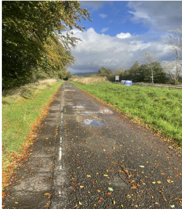
Figure 8 - Cycle track on the A74(M) A701 (source: Alistair McNay)
