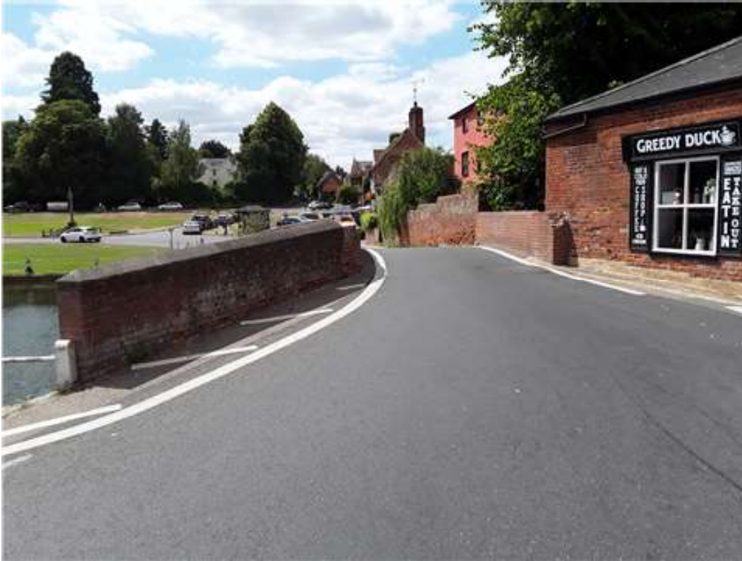
Above Structure - Facing West General View Photos
