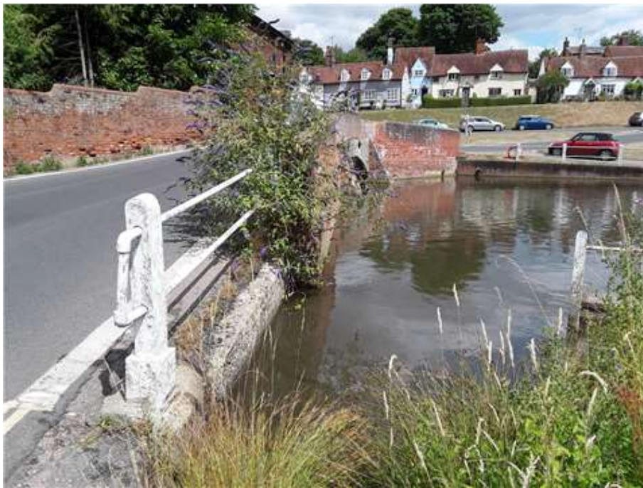
20220715_140521.jpg Upload/Link Photos to : 31 - 31/Wing walls
