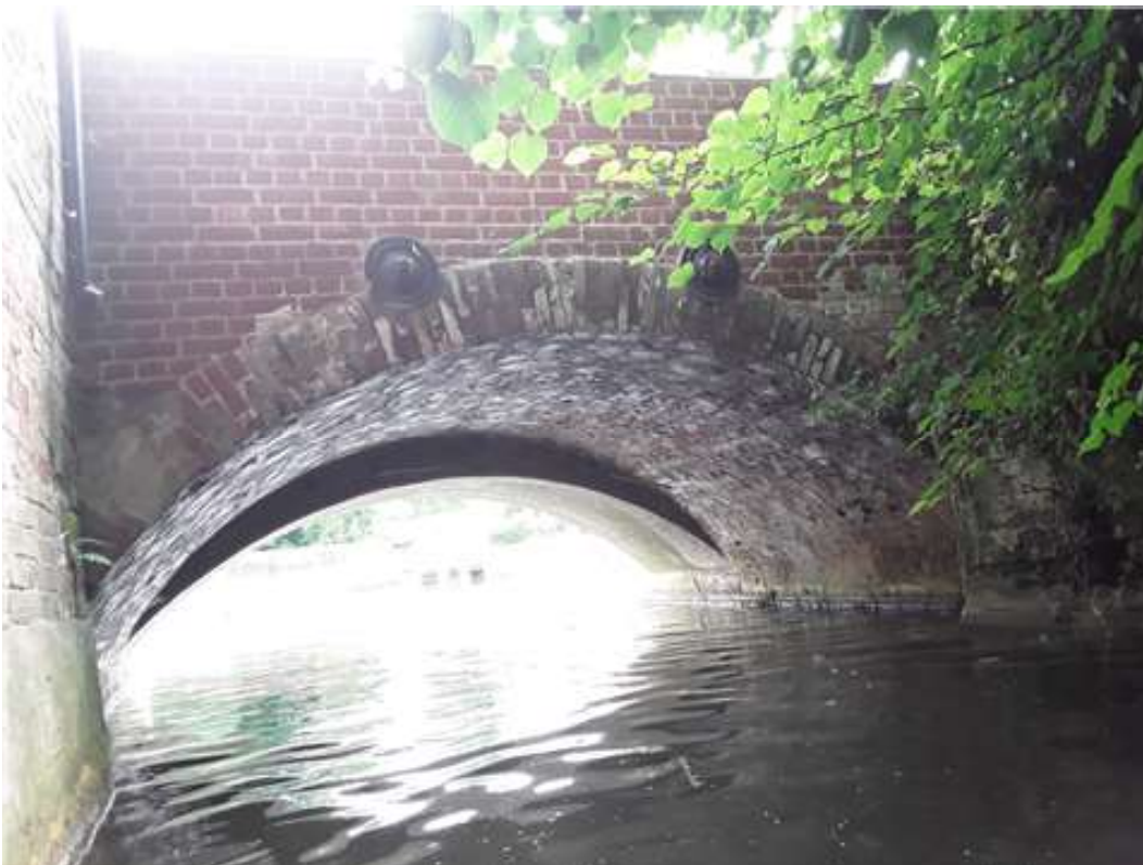
North Elevation General View Photos
