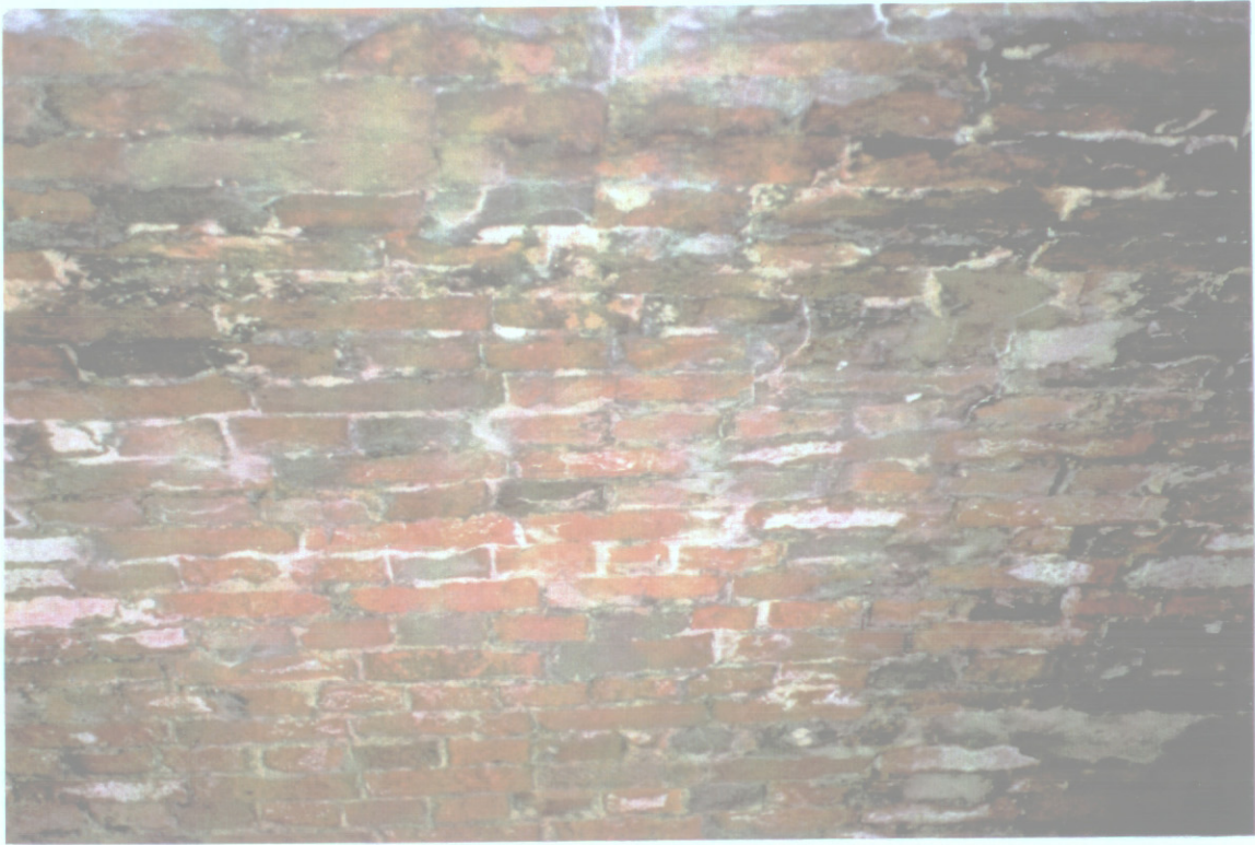
Photograph 7. Barrel brickwork.
