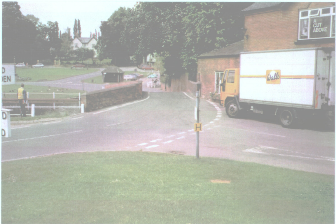
Photograph 2. Carriageway looking west.
