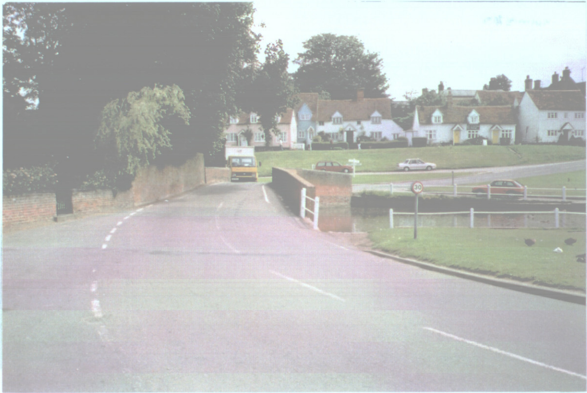
Photograph 1. Carriageway looking east.
