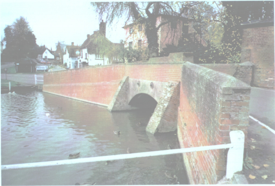
Photograph 5. Downstream parapet/wingwall.
