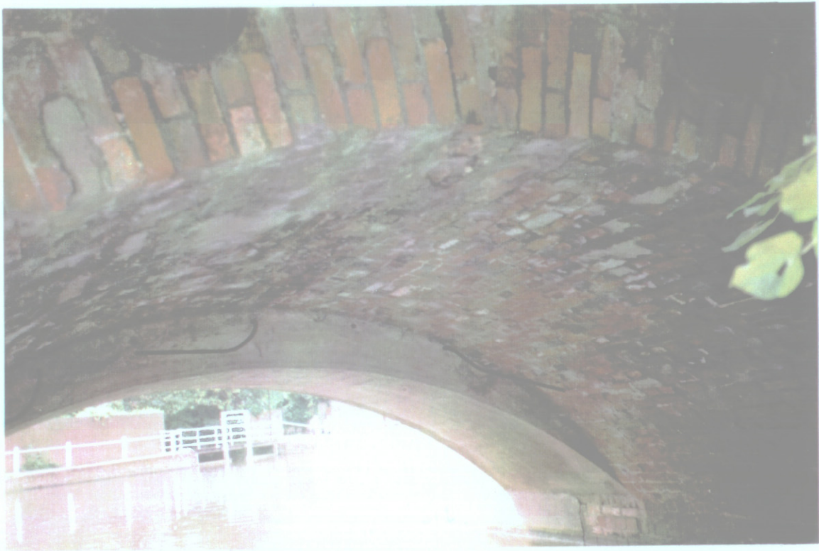
Photograph 6. Upstream brick arch.
