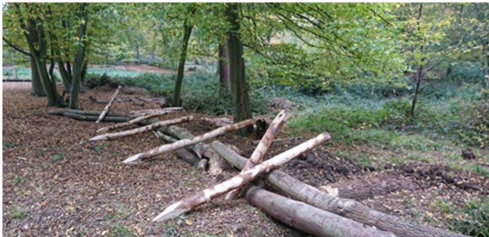
A Leaky Dam ready for Construction – photo credit: Tom Palmer / ECC
