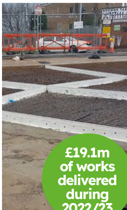
Improvement works, Wickford Station
