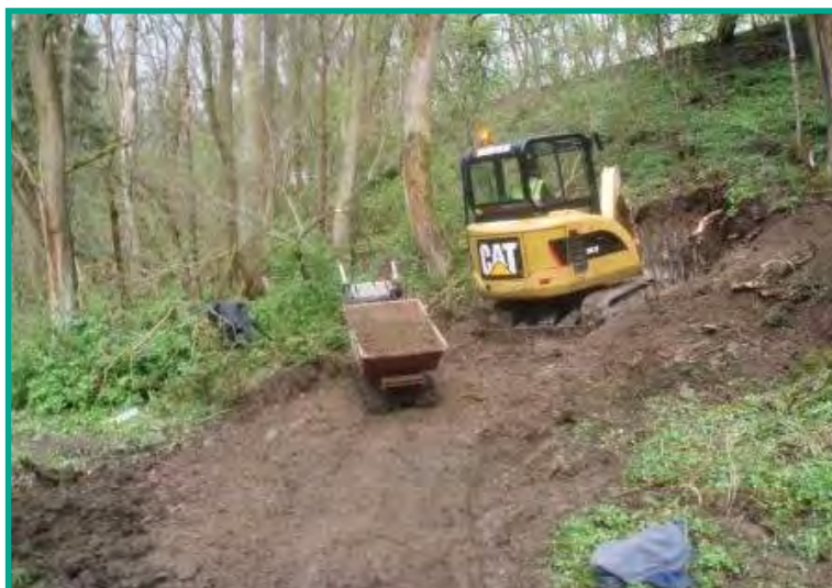
Looking for suitable materials in a borrow pit.
