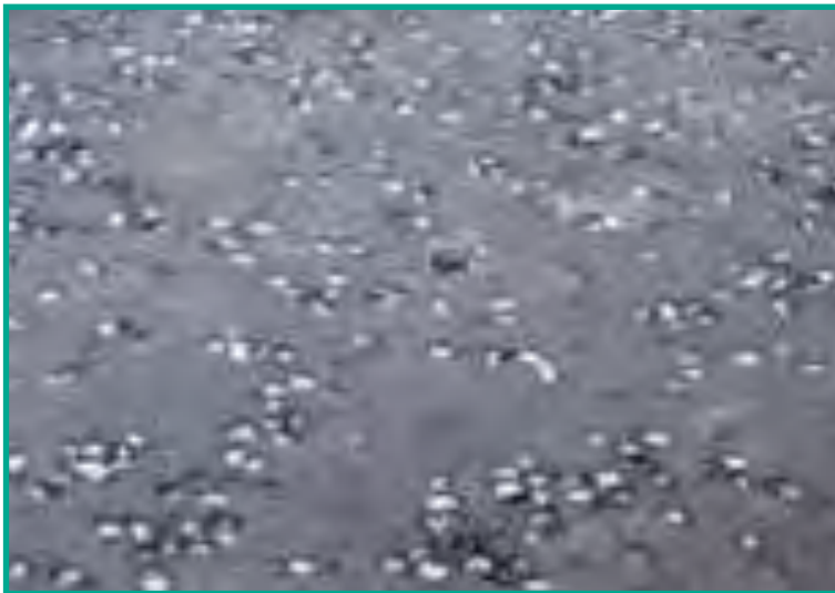
Hot rolled asphalt.
