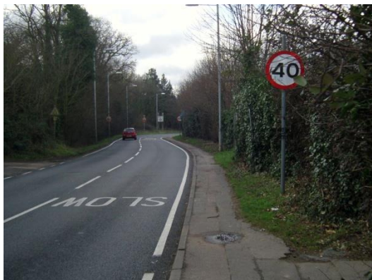
Image 5 – View from the north side looking west along Berechurch Hall Road.
